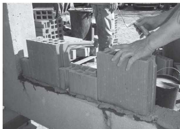
Figure 3. Construction of masonry wall.
