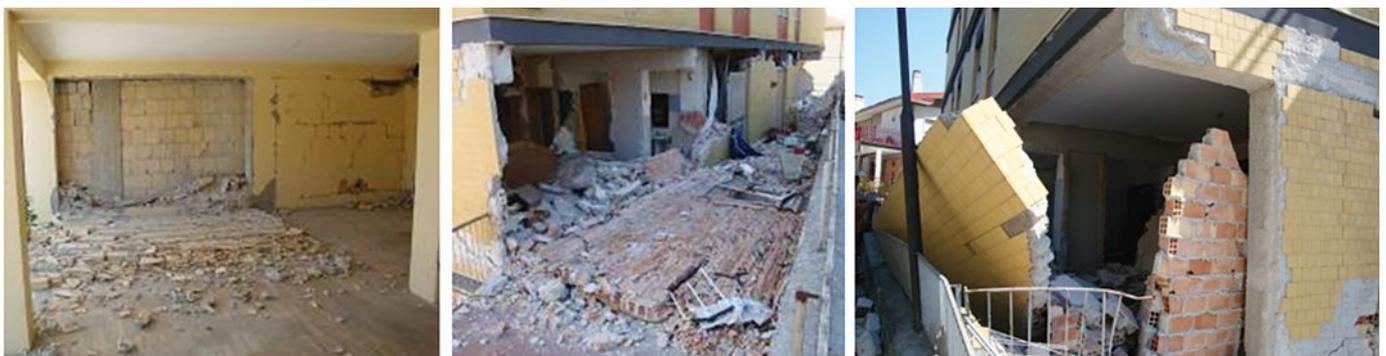
Fig. 4. Examples of seismic out-of-plane damage (L'Áquila Earthquake)
