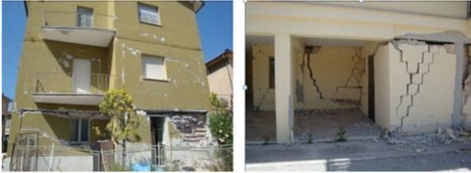
Fig. 3. Examples of seismic in-plane damage (L'Áquila Earthquake)
