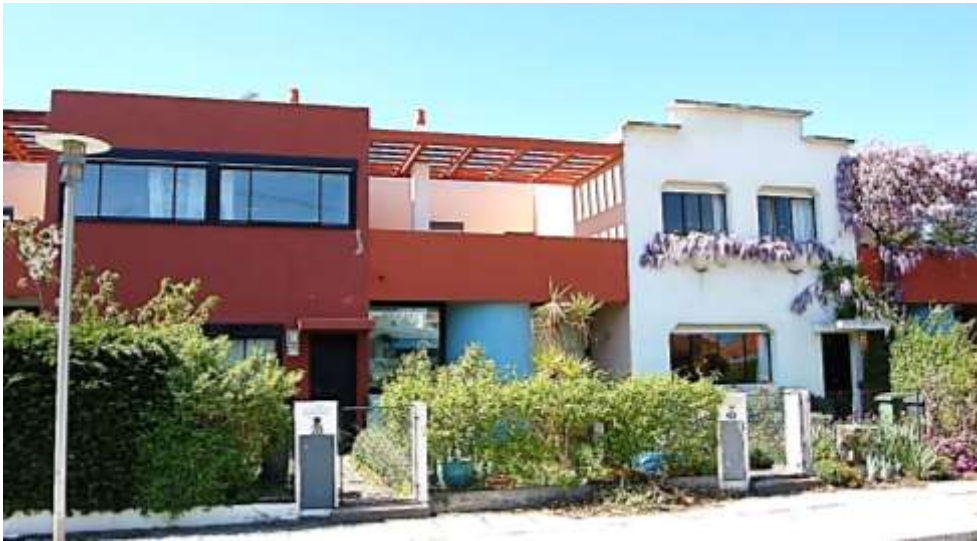
Fig. 3. Corbusier and Pierre Jeanneret, ' Quartiers Modernes Frugès ', Pessac, France, 1924-27. Image of two ' Quinconce ' houses: the one on the left was recently recovered according to the initial project; the one on the right still presents dwellers alterations (photo by the author, 2009).
