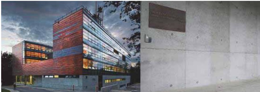
Figure 2 Photos of the entrance of Institute for Nanomaterials at TUL consisting of concrete panels which were protected by the BALCLEAN coating. To observe the self-cleaning function, only each second stream was coated, as illustrated in the picture on the right.
