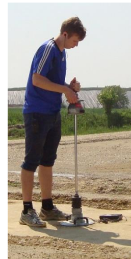
Dynamic load plate tests after each roller pass
