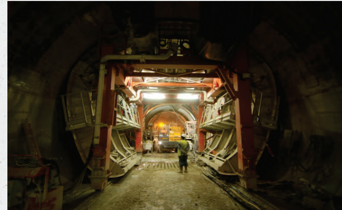
Tunnel lining formwork
