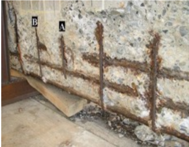
Chloride diffusion – Corrosion of steel
