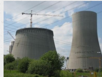
Cooling tower shell 'Hamm Westfalen', d_w = 0.3 m
