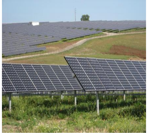
A Panoramic Image of a Photovoltaic Farm:
