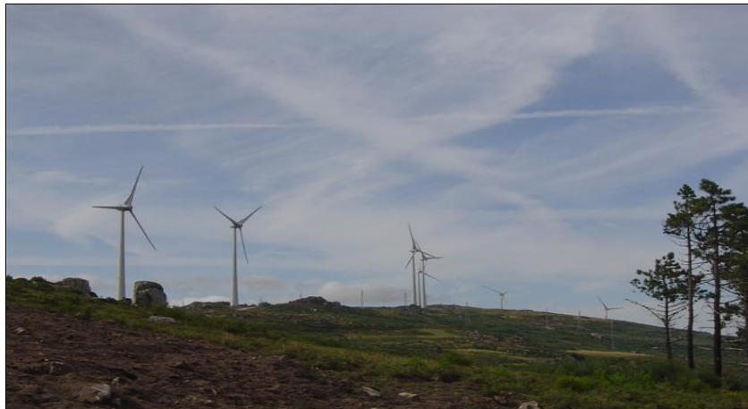
Figure III.28: Panoramic Image of Negrelo & Guilhado Wind Farm
