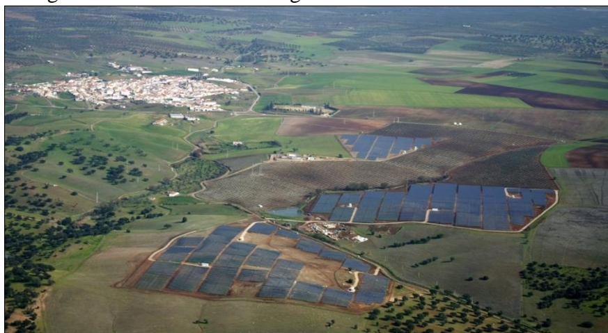
Figure III.32: Panoramic Image of Hércules Photovoltaic Farm
