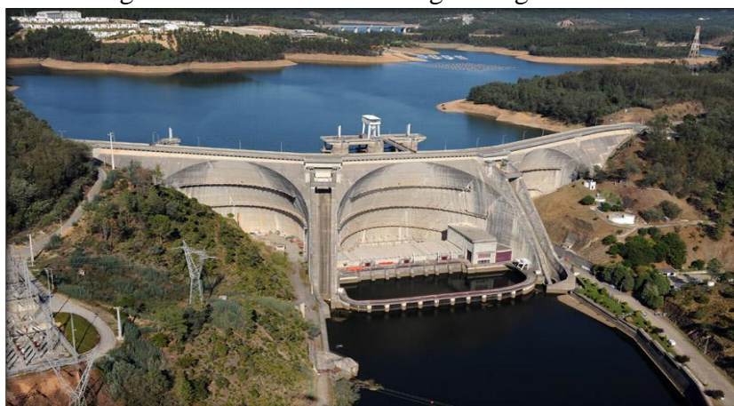
Figure III.17: Panoramic Image of Aguieira Dam
