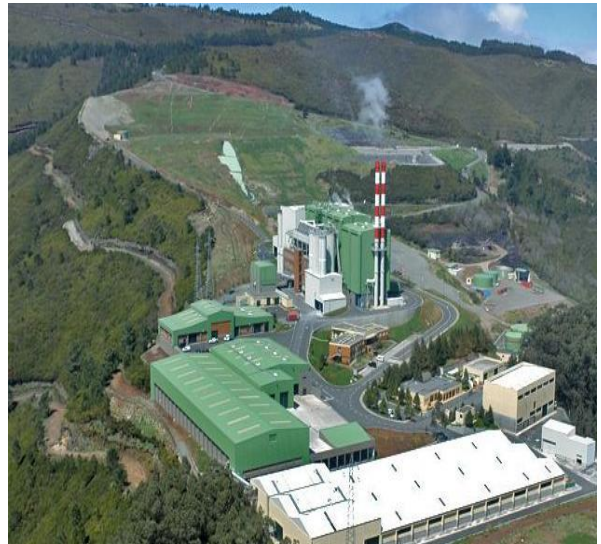
A Panoramic Image of a Biomass Power Plant:
