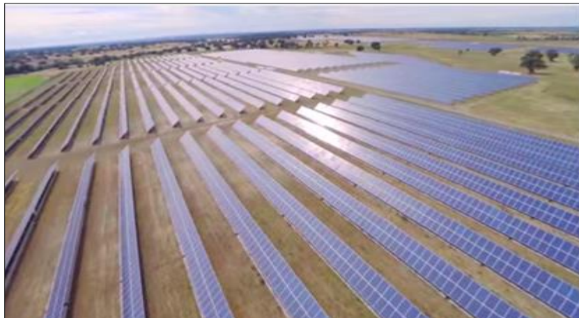
Figure III.36: Panoramic Image of Ferreira do Alentejo Photovoltaic Farms
