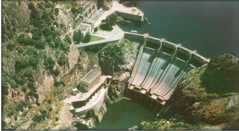
Figure III. 11: Panoramic Image of Picote Dam
