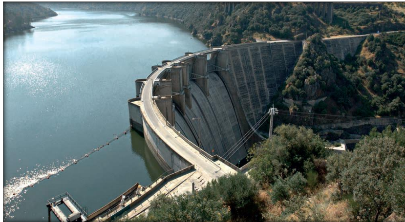
Figure III.14: Panoramic Image of Bemposta Dam
