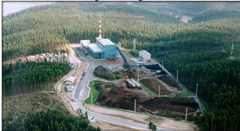
Figure III.40: Panoramic Image of Mortágua Forest Biomass Power Plant
