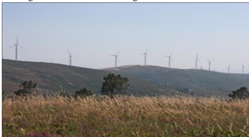
Figure III.26: Panoramic Image of Lousã II Wind Farm
