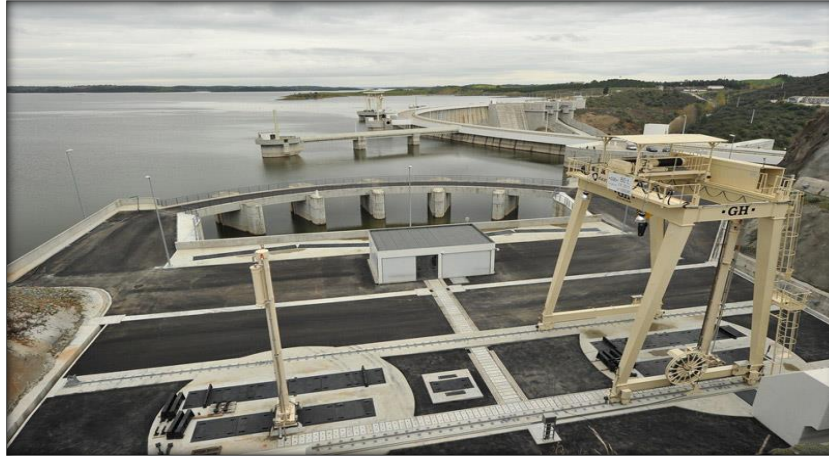
Figure III.20: Panoramic Image of Alqueva II Plant
