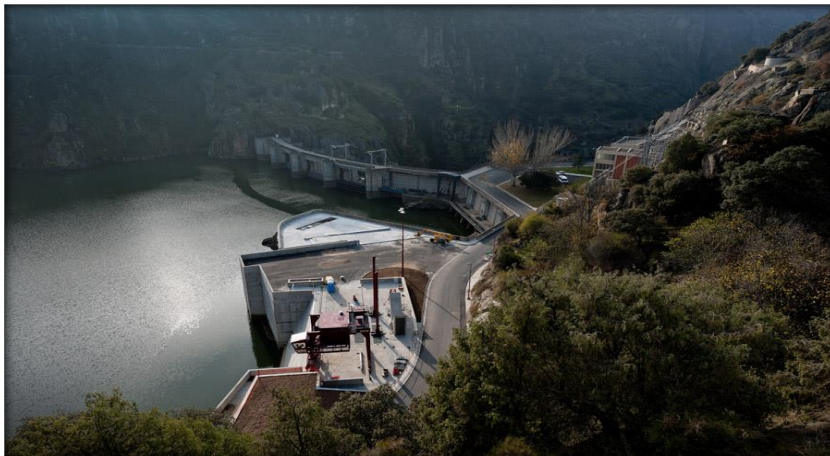
Figure III.12: Panoramic Image of Picote II Plant
