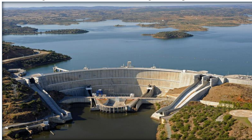
Figure III.19: Panoramic Image of Alqueva Dam
