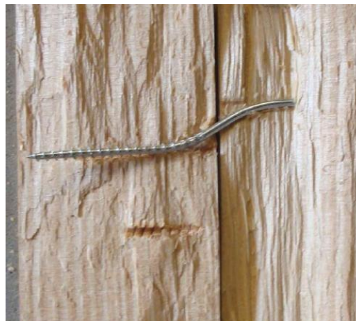
Figure 15: Failure mode of the tested connections, where is visible the local crushing of timber near the connection and the bending of the screw.
