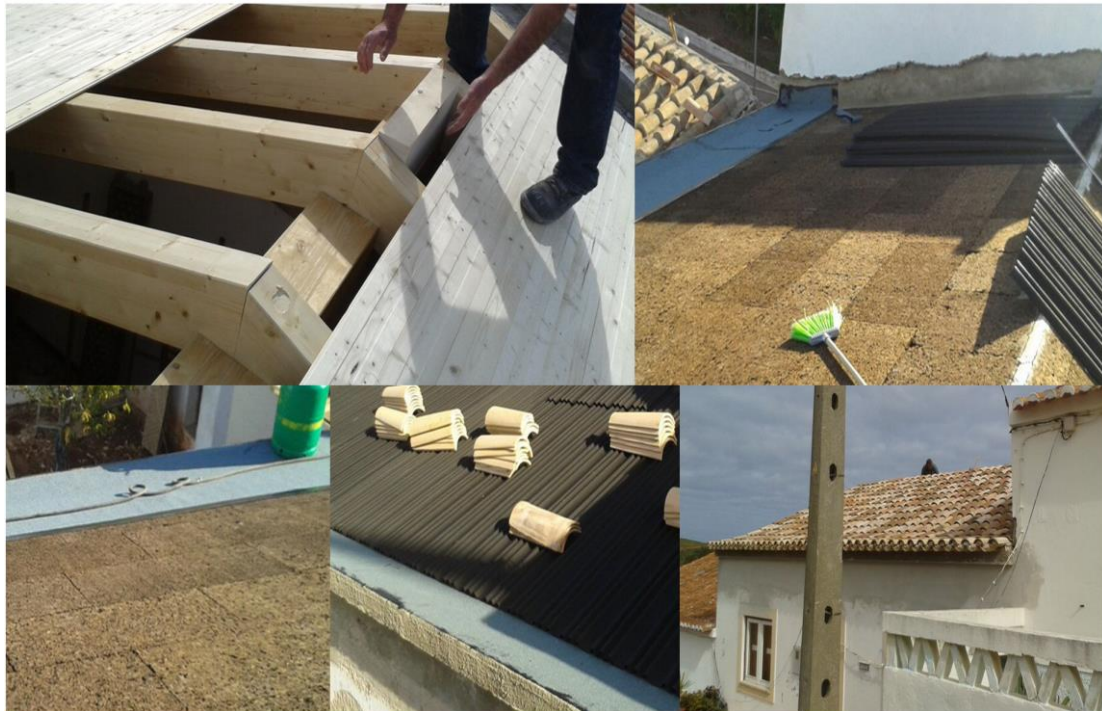
Figure 8 - Installation of insulation on ceiling during its renovation (Lima & Rocha, 2015)
