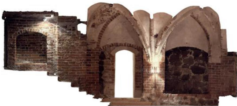
Figure 18 - Room in the Museum Centre of Turkey (COBIM, 2012b)
