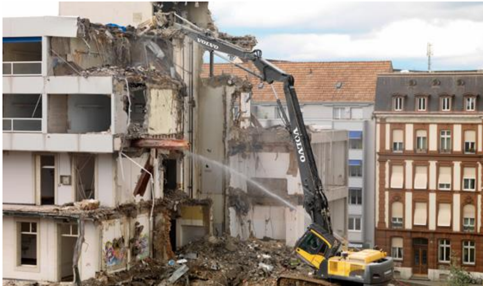
Figure 4 - Building being demolished by pneumatic machine (Volvo, 2010)
