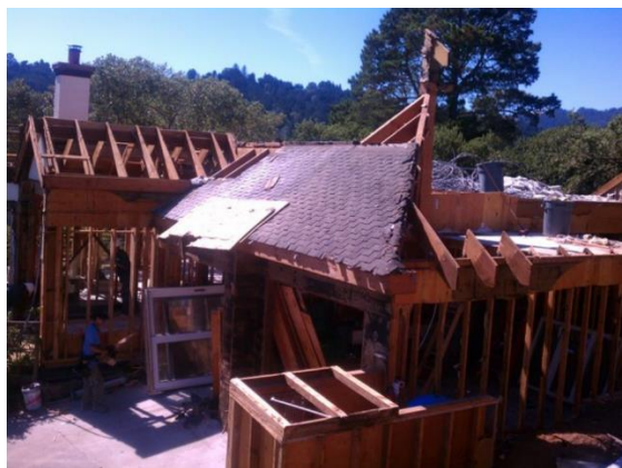
Figure 3 - Disassembling parts of a building (Hurricane Hauling & Demolition, 2012)
