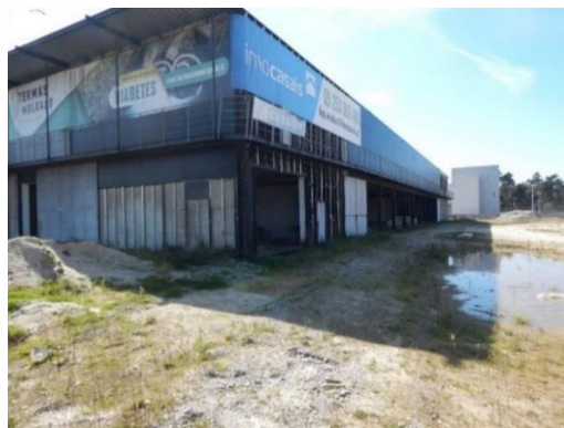
Figure 38 - Itarion photo - Back Façade
