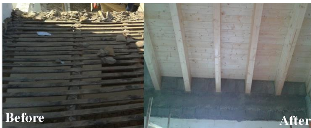
Figure 9 - Before and after refurbishment (Lima & Rocha, 2015)
