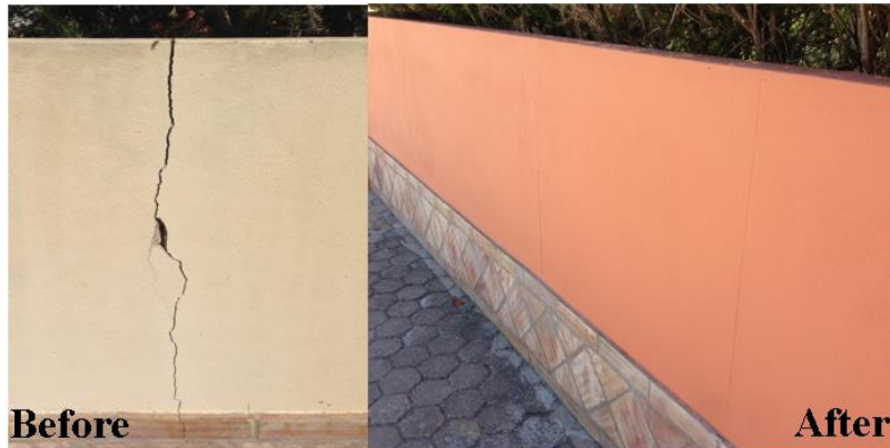
Figure 5 - Before and after renovation (Lima & Rocha, 2015)
