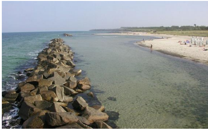
Figure 2.4- Breakwaters in front of a public beach [11].
