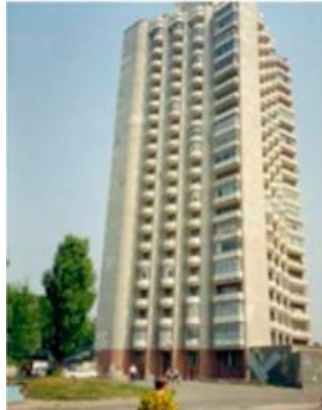
Figure 2. 19- The first residential building made of alkali-activated cement concrete without any OPC. (20-storey residential building, Lipetsk, Russian Federation, 1987–1989) [44].
