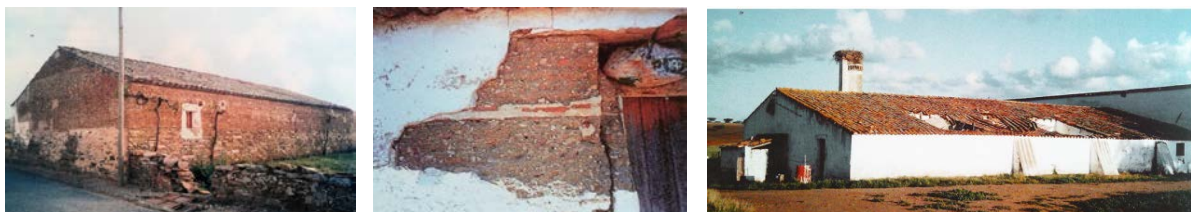
Figure 3: (left) Stone base course [20]; (middle) brick masonry horizontal course within rammed earth walls [20]; chimney [20]
