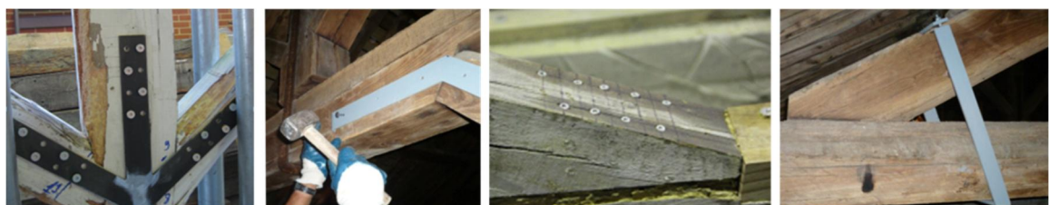
Fig. 17 – Contemporary strengthening interventions on notched joints reproducing old techniques.
