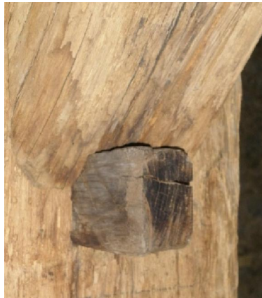
Fig. 10 – Wooden wedge to ensure the contact between the tenon and the mortise.
