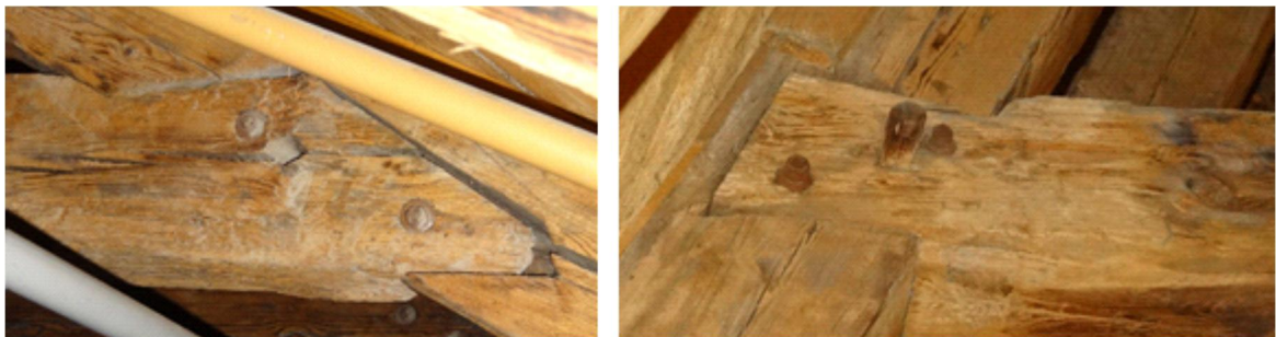
Fig. 21 – Traditional reinforcement of dovetail-lap joints under tension loads by adding wooden dowels
