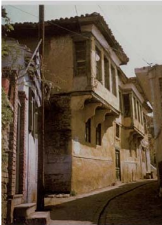
Figure 1. Building in Epimenidou Street, Thessaloniki, picture by: Michael Nomikos
