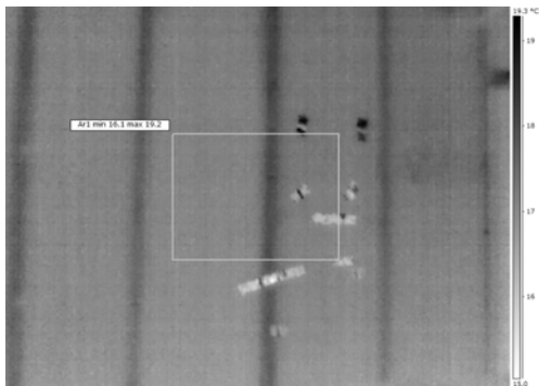
Figure 6. Infrared thermal image of a LSF wall without ETICS (external surface).
