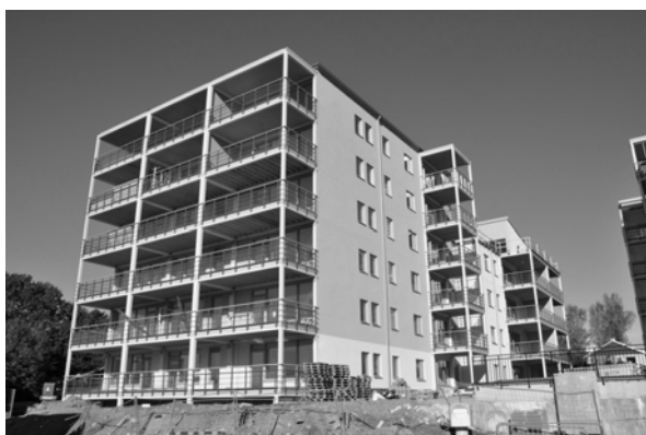
Figure 2-1 Trä8 in Gothenburg Sweden, (Photo Per Skogstad)
