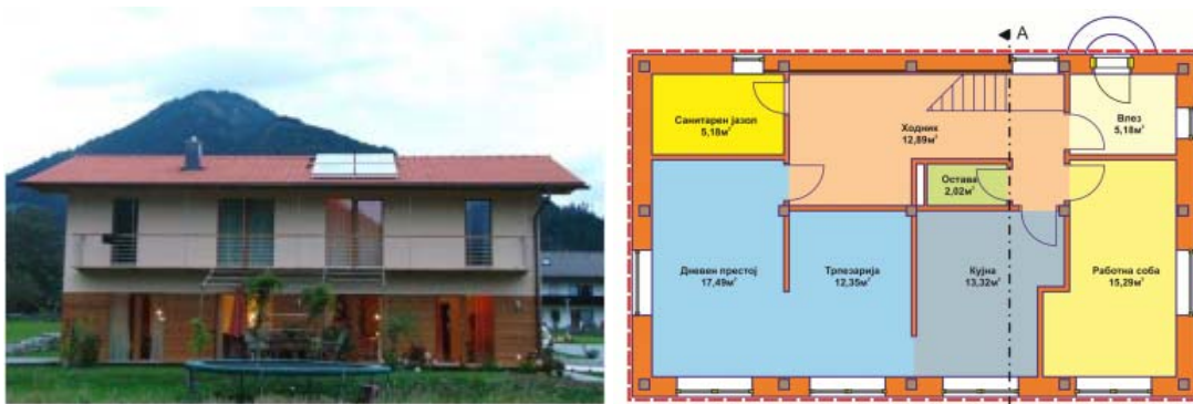
Figure 2. Passive house designed by Franz Freundorfer
