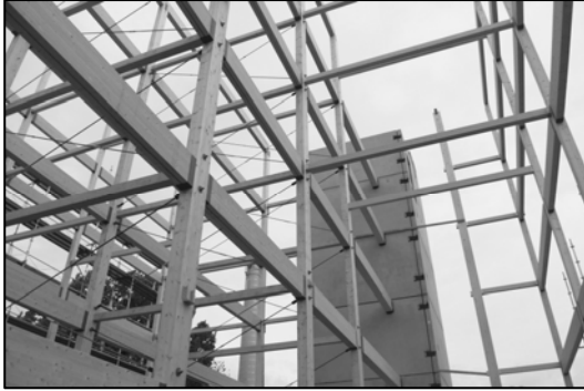
Figure 2-2 Gluelam beams and posts in the building (Photo: Per Skogstad)
