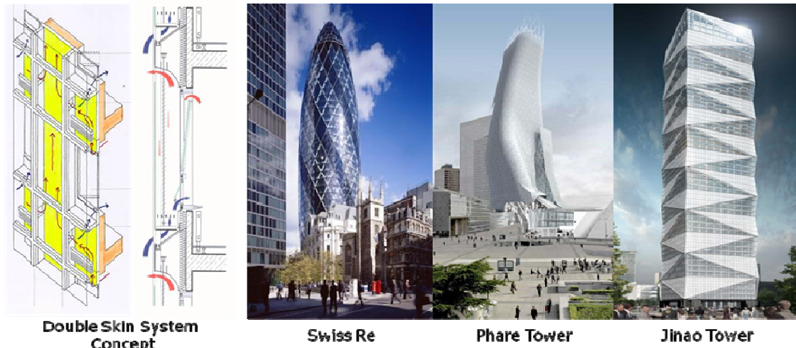
Figure 13. Double Skin System design Concept and Cases
