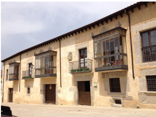
Figure 5. Ironwork Sunspace in Ledesma , Spain
