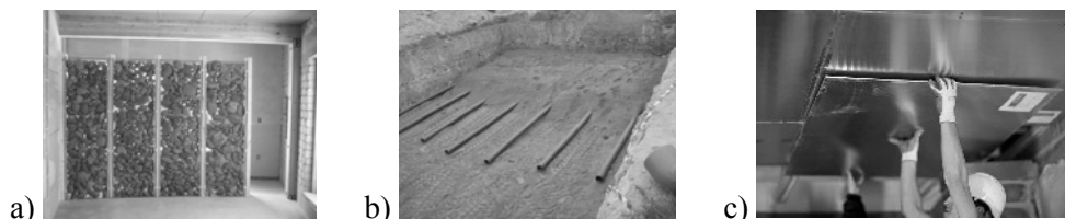
Figure 3. Thermal inertia improvement: a) wall filled with stones (Detect Energy 2013); b) ground heat exchanger air circulation pipes; c) PCM panels (DuPont 2013).
