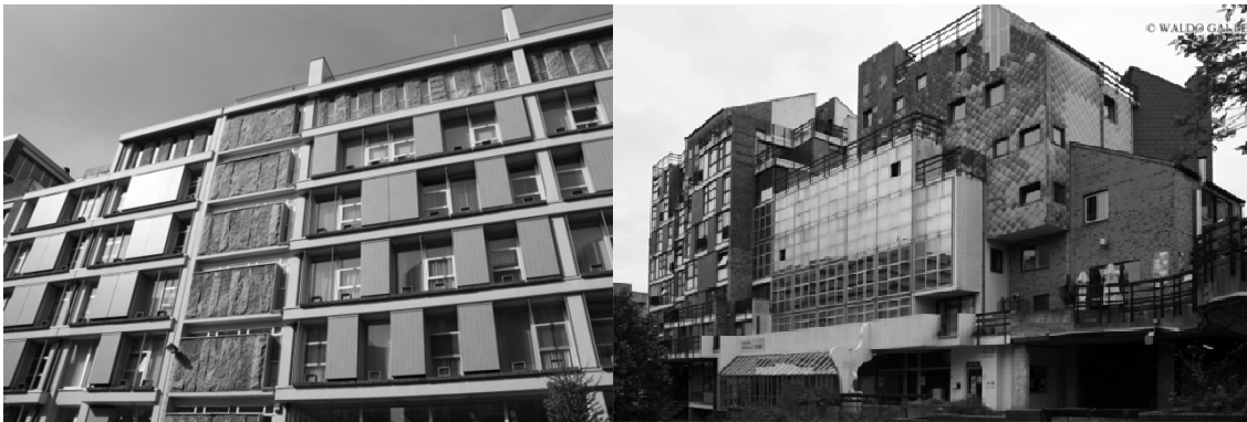
Figure 3. The analysis of the HBK bank office (left) and La Mémé (right) illustrated the applicability of the time-dependent design aspects that were derived from literature. Photos by the first author.
