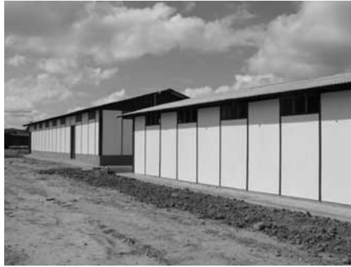
Figure 1. OSB prefabricated temporary facilities. Source: http://www.lpbrasil.com.br/aplicacoes/
