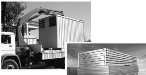
Figure 7. Containers transported either assembled or disassembled.
