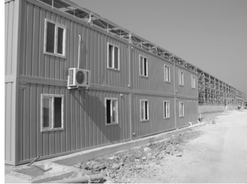
Figure 6. External view of metal container with air conditioning.
