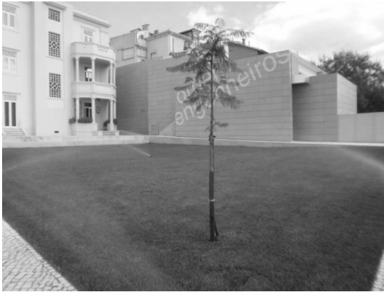
Figure 1. The sprinkler system
