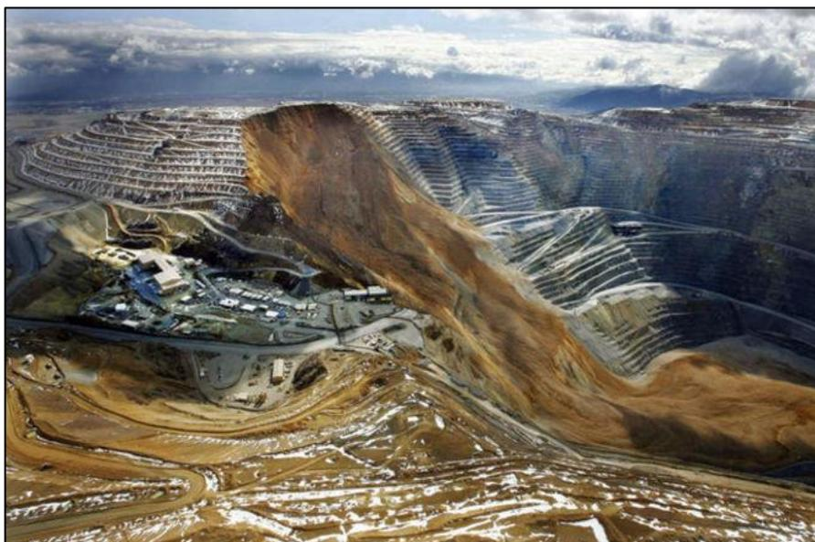
Figura 2.2 – Rotura de talude da Mina de Bingham Canyon, Kennecott Utah (USA) (adaptado de Caldwell, 2013)
