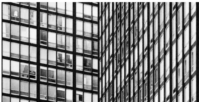
Figure 2.12. Lake Shore Drive 860 facades.
