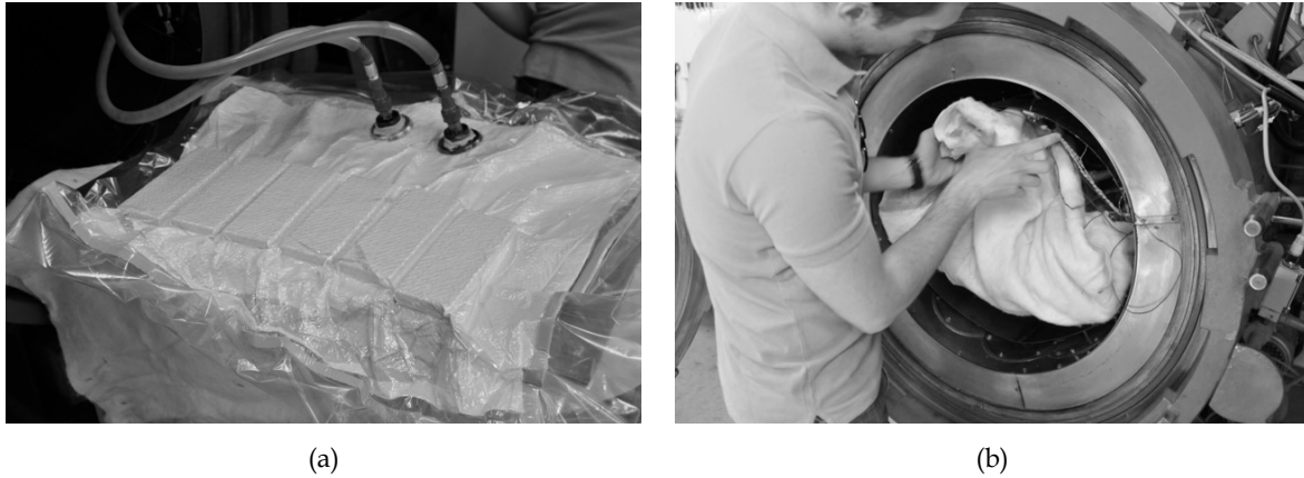
Figure 6.13. Connection of the bag to the vacuum pump (a) and introduction of the bag inside the autoclave (b)
