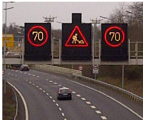
Figure 2: Variable speed limits digital signs (By GilPe, Own work, CC-BY-SA-3.0, http://creativecommons.org/licenses/by-sa/3.0 , via Wikimedia Commons)
