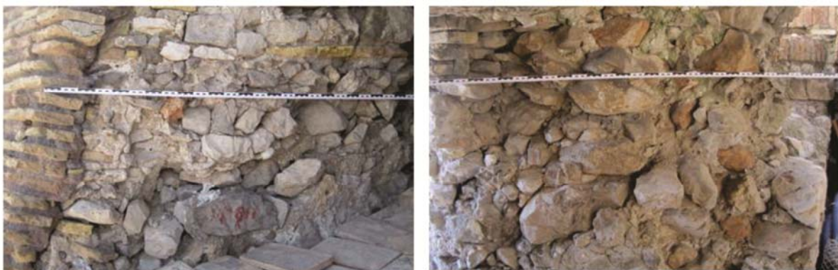
Figure 4. Visual inspection: wall cross section.
