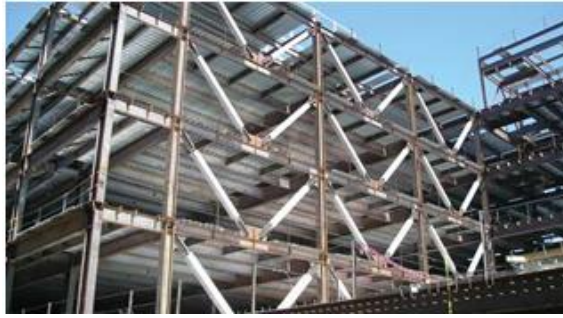
Figure 8 - Bracing systems (adapted from [23])
