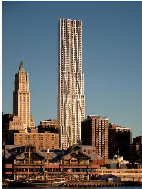
Figure 39 - Eight Spruce Street Building, the tallest residential building (adapted from [142])
