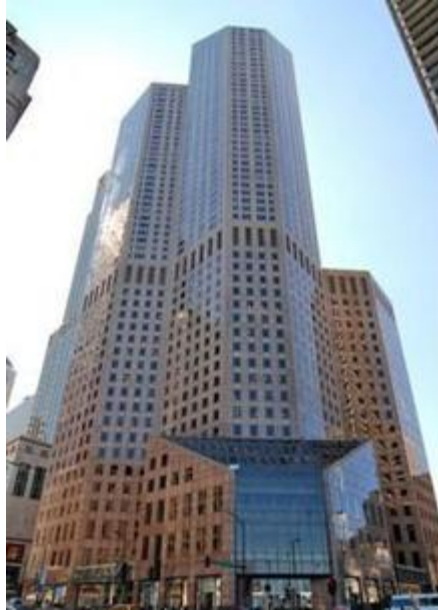
Figure 18 - One Magnificent Mile Bundled Tube System (adapted from [31])
