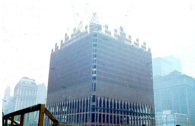
Figure 14 - Columns merging at the entrance level at World Trade Center (adapted from [28])
