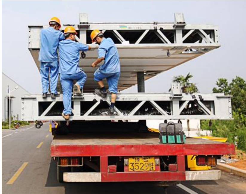
Figure 43 - Truck Transport of a Modular House (adapted from [161])
