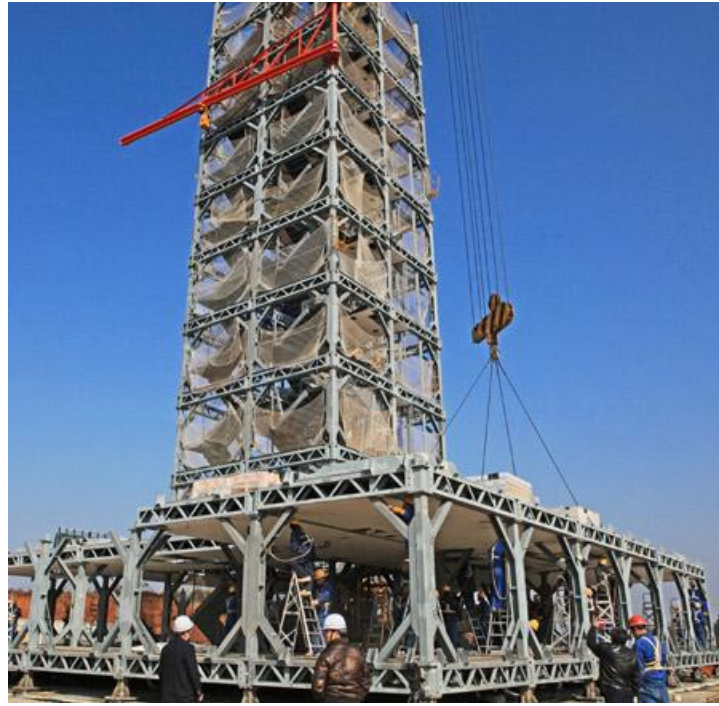
Figure 54 - Hotel T30 steel construction(adapted from [171])
