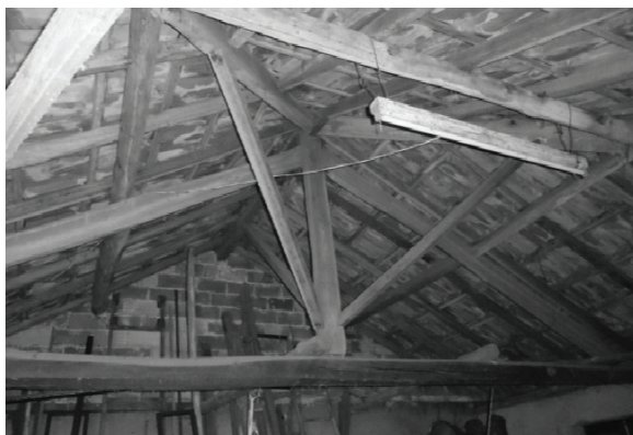
Fig. 16. Covering Structurally Supported by Wood Trusses
