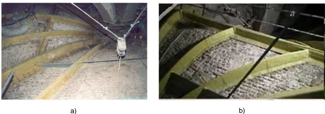
Fig. 2.5. Use of suspension solution in Basilica of Saint Francisco di Assisi [11].
