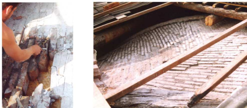
Fig. 2.7. Reconstruction of a part of a soldier masonry vault of the St. Fermo Church in Verona, Italy [14].
