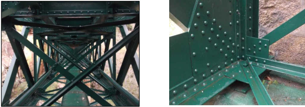
Figure 2 Images of the on-site geometry survey [3]
