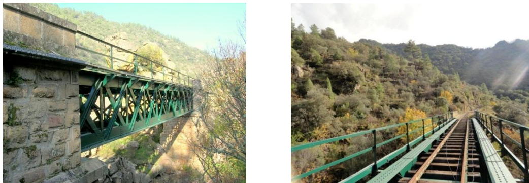
Figure 1 The Paradela Bridge [2]
