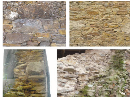
Figure 12. Examples of regular and irregular masonry. Examples of masonry's section and core. (Credits: C.E. Barroso et al.).
