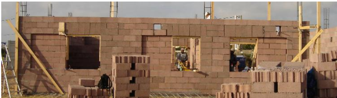
Figure 11. Example of modern confined masonry under construction.
