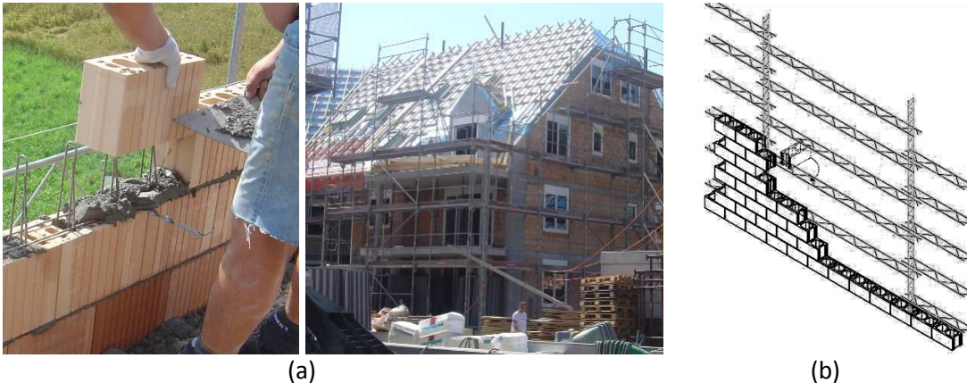
Figure 10. Modern reinforced masonry solutions: (a) Switzerland; (b) Spain for infills.
