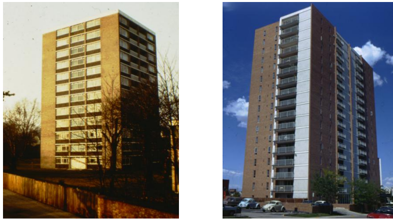
Figure 2. Modern (unreinforced) masonry high rise buildings, designed for compression / shear.
