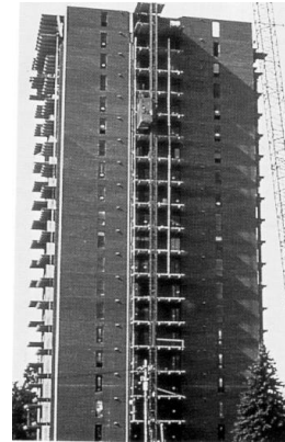
Fig. 4. Modern (reinforced) masonry in high rise buildings up to 30 stories, designed for compression, shear and tension.
