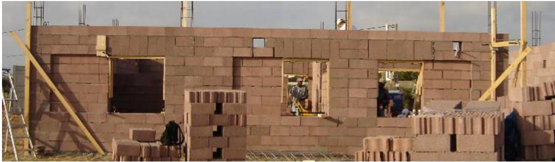
Fig. 11. Example of modern confined masonry under construction.
