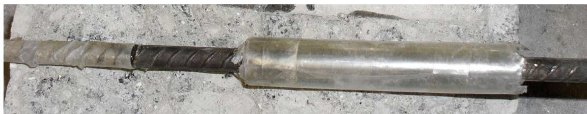
Figura 6.3: Jacketing of the steel bar with a plastic tube to obtain the unbounded length.
