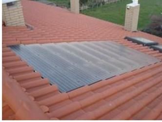
Figure 5 – Photovoltaic tiles (Enat – Energias Naturais, 2012).
