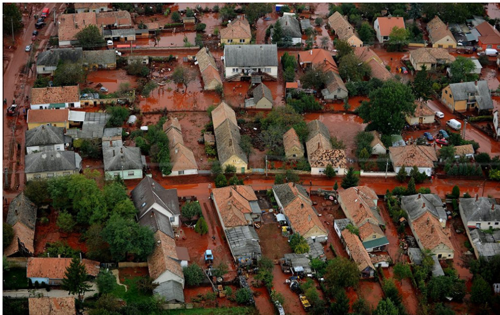
Fig. 1. One million cubic meters toxic red mud spilled into Kolontar village (Hungary) after aluminium mine tailing collapse. (For interpretation of the references to colour in this figure legend, the reader is referred to the web version of this article.)
