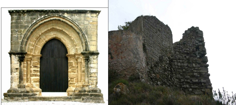
Fig. 1. Traditional buildings with load bearing masonry: (a) vernacular masonry buildings with granite; (b) historical and vernacular construction in sandstone
