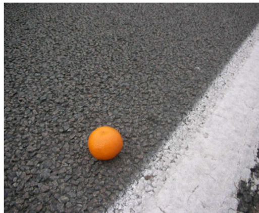
Fig. 17. Single layer porous asphalt (0/14).
