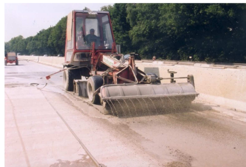
Fig. 24. “Chemical washing” of cement concrete: immediately after the laying of the concrete, a retarder is sprayed on it and it is covered with a plastic foil (left hand side). The unhardened cement of the upper layer is removed after 12 – 24 h with a brush and water (right hand side).
