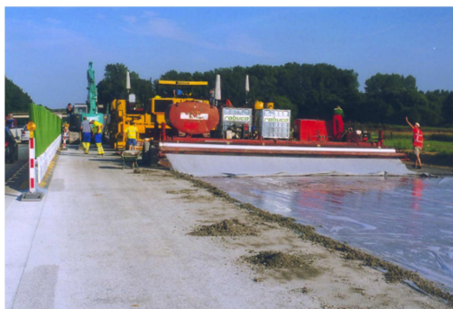
Fig. 24. “Chemical washing” of cement concrete: immediately after the laying of the concrete, a retarder is sprayed on it and it is covered with a plastic foil (left hand side). The unhardened cement of the upper layer is removed after 12 – 24 h with a brush and water (right hand side).
