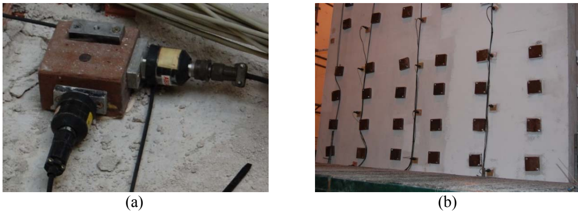
Figure 5: Instrumentation of the model using accelerometers: (a) in the concrete structure (corner of the slab measuring transversal directions); (b) infill walls (South wall, storey 1)
