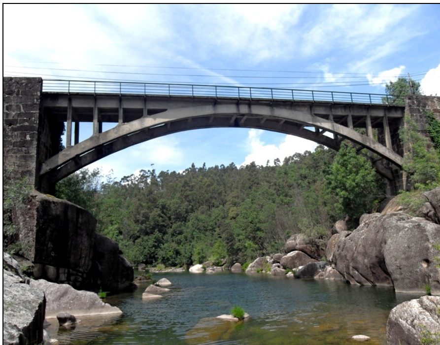
Fig. 2 View of the Bôco Bridge revealing its current state
