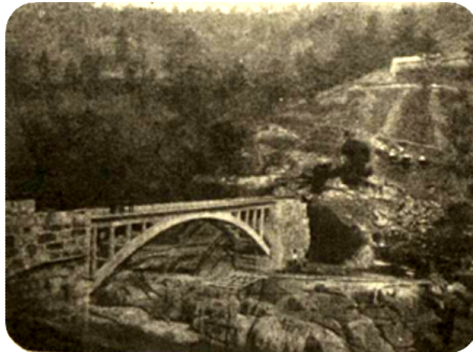
Fig. 1 Photo of the bridge after its construction [1]
