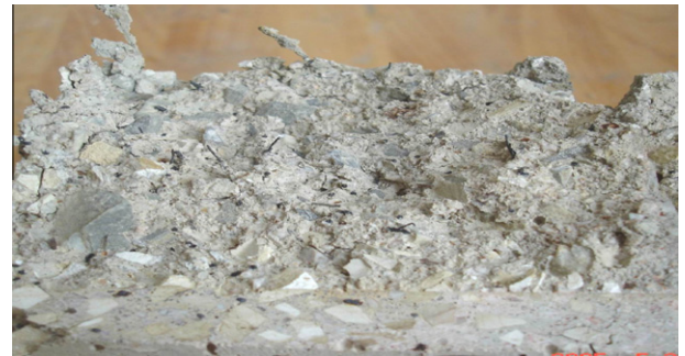
Fig. 13b. Failure pattern of SF55 after 900 °C.
