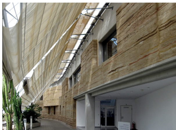
Fig. 7. Rammed earth wall, Hospital of Feldkirch, Austria [10].
