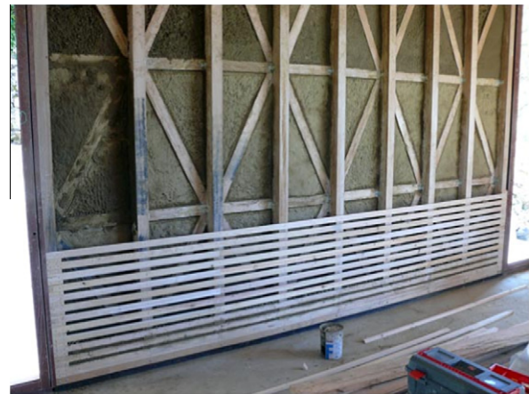
Fig. 1. Hybrid earthen wall system.
