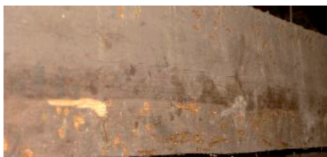
Figure 2. Emergence holes over the surface of sapwood.
