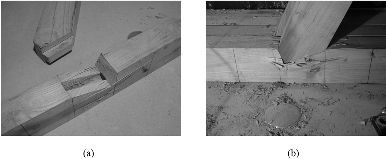
Figure 7.12 – Typical experimental failure patterns observed: (a) joint collapsed in compression, with damage localized at the toe, and (b) joint collapsed in compression, with uniform distribution of damage.
