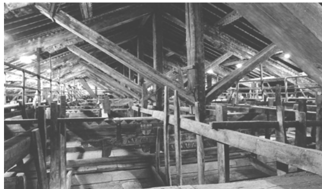
Figure 1.1 – The complexity and extraordinary space between roof (timber carpentry of the XIII c.) and false ceiling (timber carpentry of the XVIII c.) of the Saint Mark's church in Florence, Italy.
