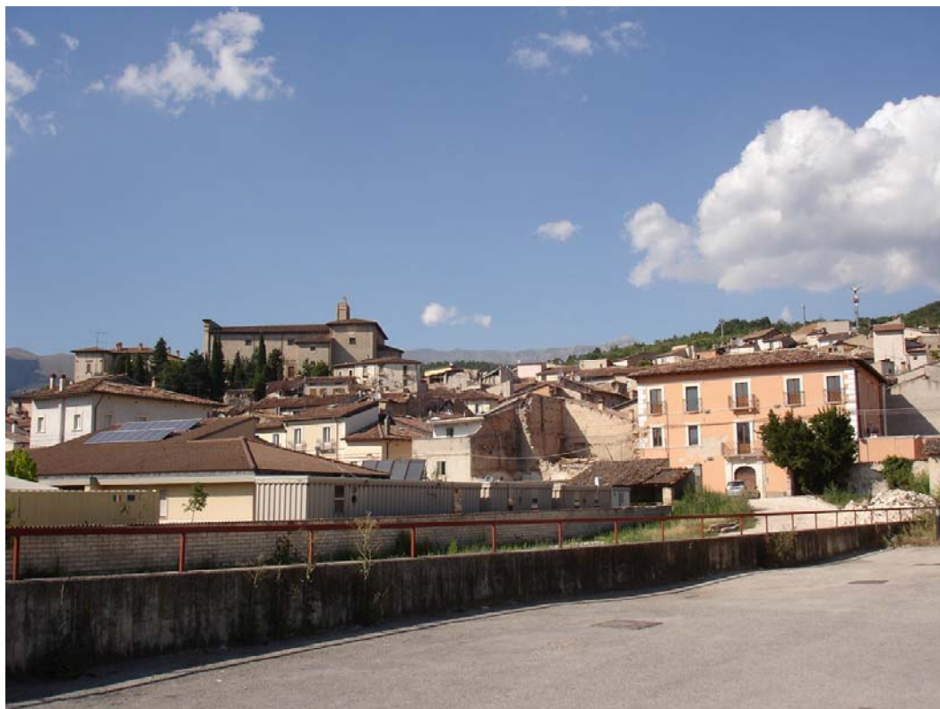
Fig. 2.4 Historical centre of Paganica – Lower view.
