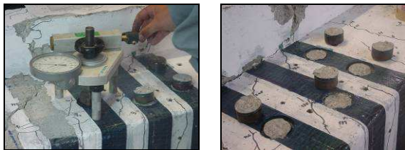
Fig. 5 – Ensaios de pull-off.
